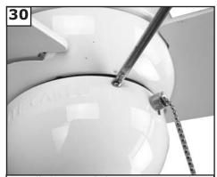
Install the switch housing using the 3 screws previously removed.
